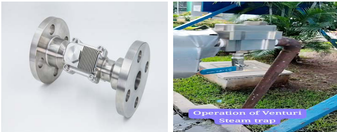
Figure 28 Image of Venturi Steam trap and its actual installation
