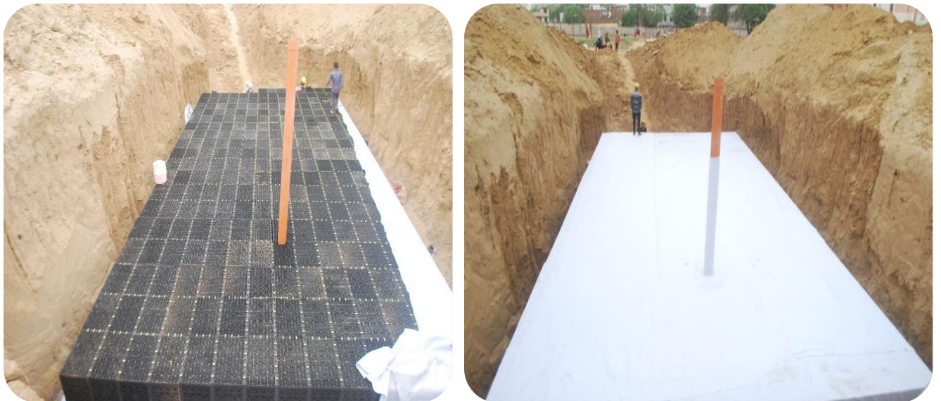
Figure 21: Actual site installations
