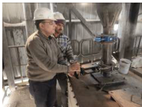
Figure 11 Installation of feeding system for Oxy-booster
