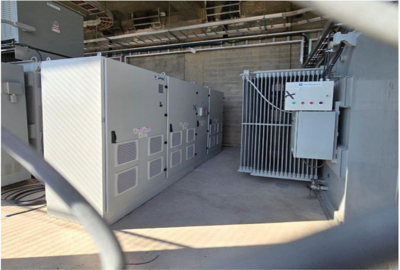
Figure 22 Photos of installation
