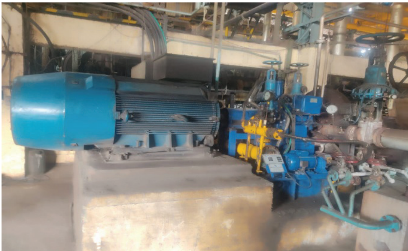
Figure 8 Back Pressure Turbine
